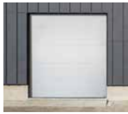
REPAIRED DOOR WITH AMARR 2747 REPLACEMENT SECTION
